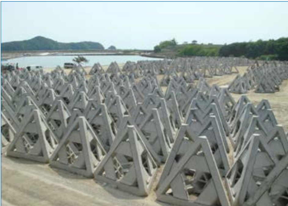
Pyramid-style artificial reefs designed for demersal reef fish, Incheon South Korea.
